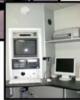
Operator Control Room
