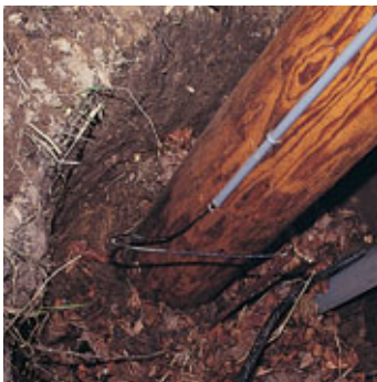
Traffic Signal Base Safely expose electrical lines for quick repairs.
